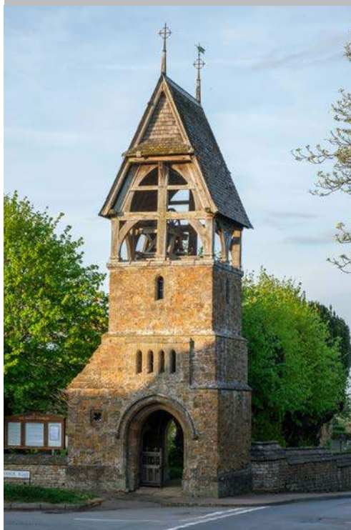
Bell tower lychgate - Great Bourton Repairs to lychgate £7000
